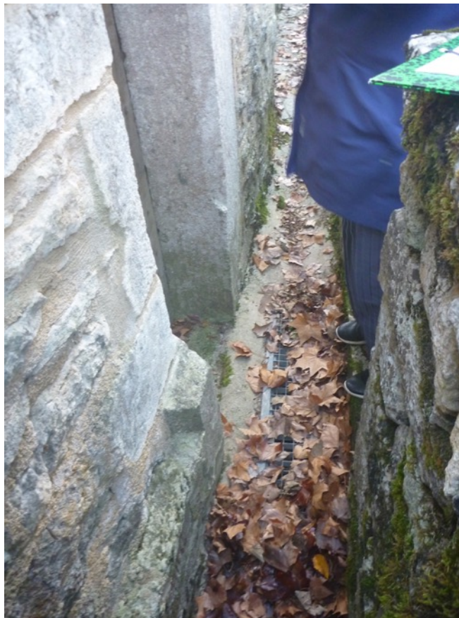
Figure 4: View towards the west of the ground around the north door with the narrow gap between the wall of the chapel (left) and the retaining wall (right). Note the plinth courses on the east side of the door and the absence of plinth courses on the west side.
