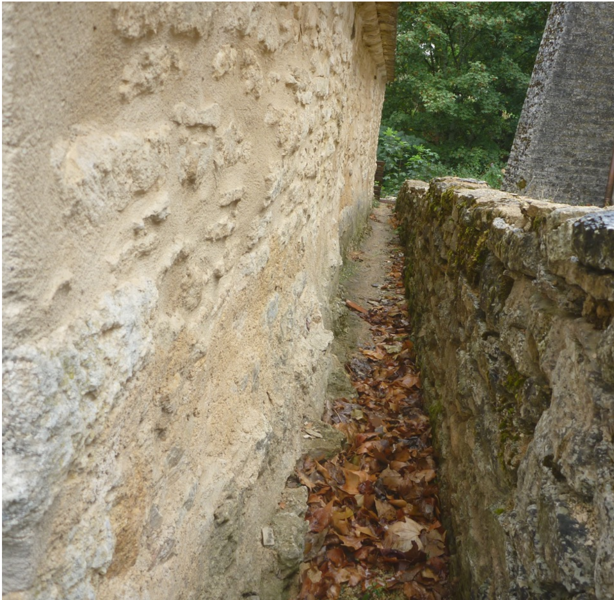
Figure 12: View along the south wall towards the east. Note the bulge distinguished by rough stone at the bottom and curve inward from there of all but the topmost courses.
